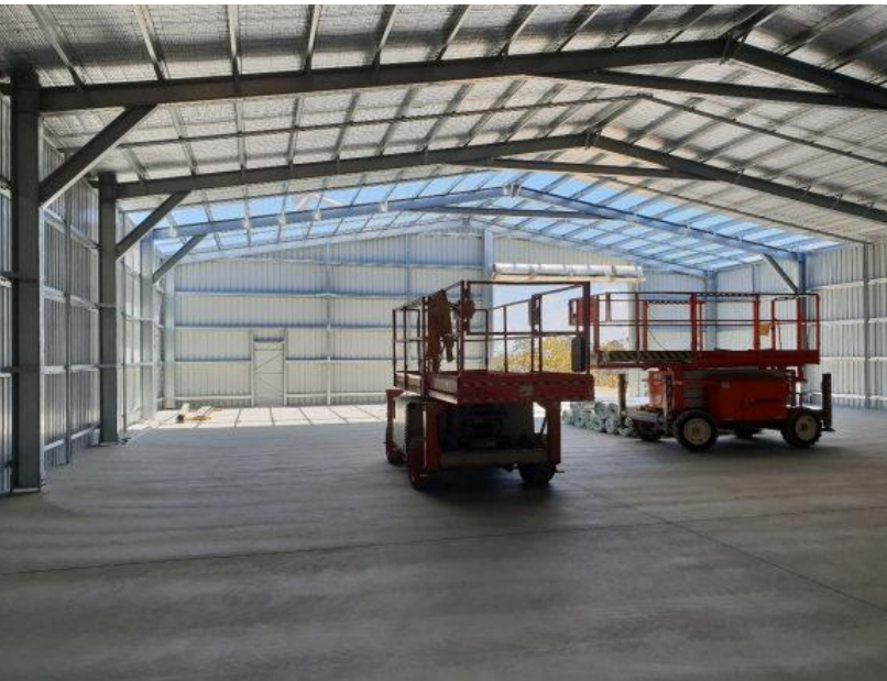
Completion of the on-site maintenance and storage shed
