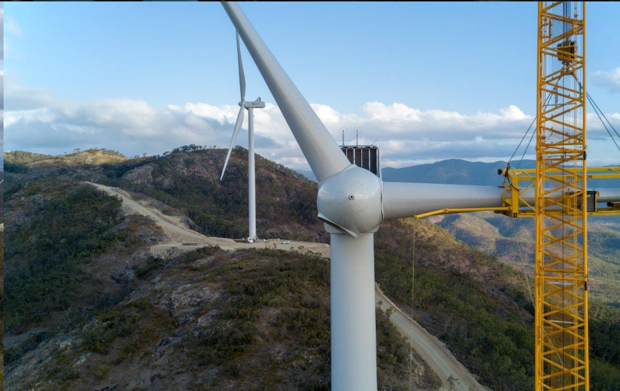
Installation of the blades on the last of the 53 wind turbines at Mount Emerald wind farm
