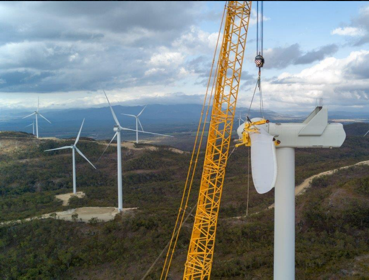
Installation of the blades on the last of the 53 wind turbines at Mount Emerald wind farm
