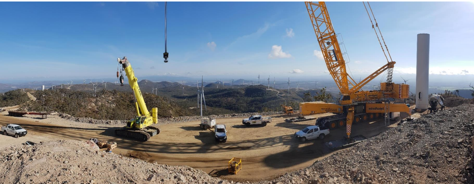
Installation works at WTG 33 looking north-west
