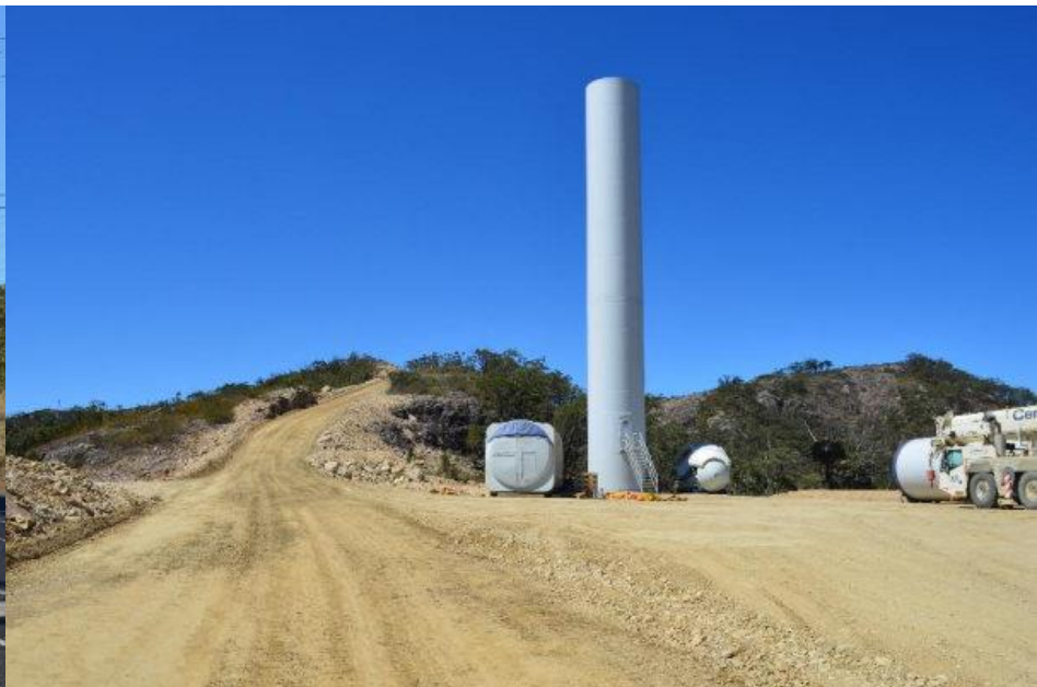
Partial install at WTG31
