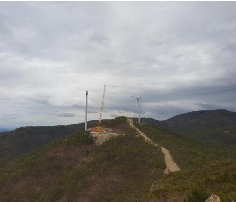
Install at WTG 20
