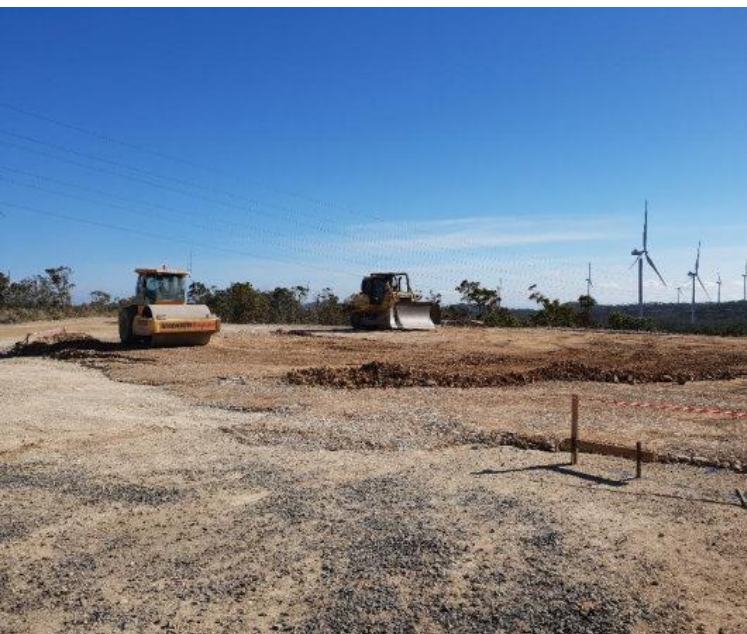
Preparation of pad for maintenance building
