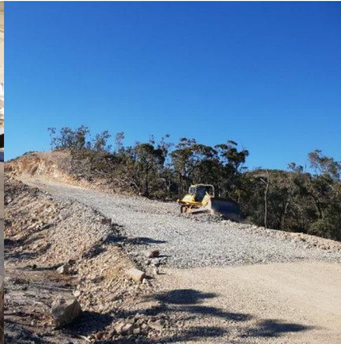
Roadworks to WTG33
