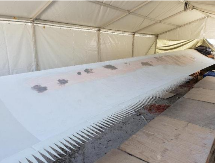
Minor repairs to blade before install
