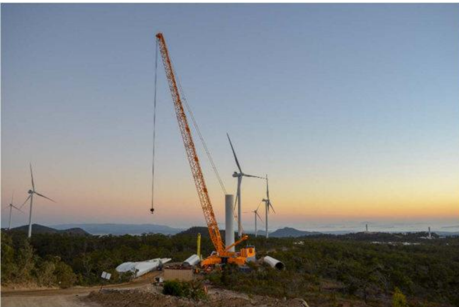
Installation at WTG14
