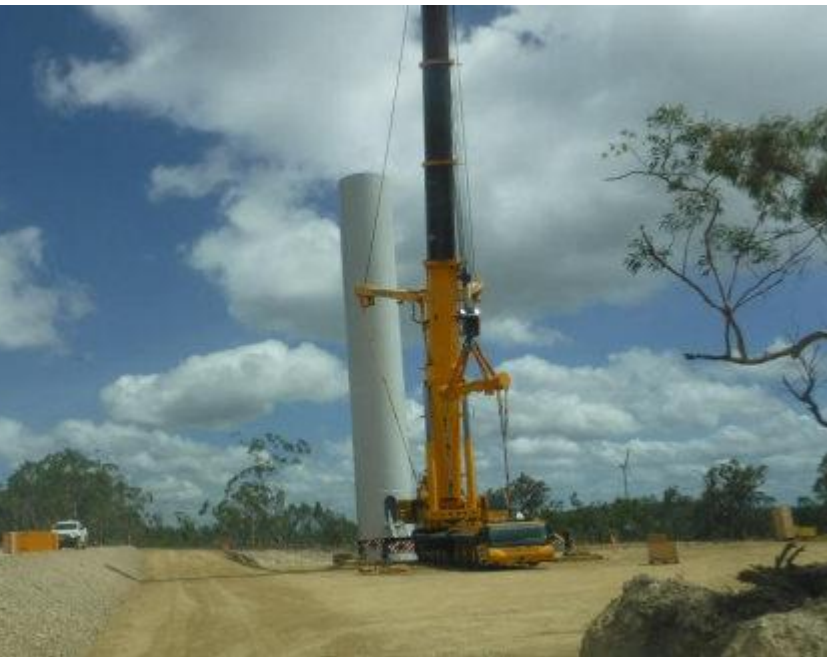
Base and mid-section installation at WTG 37
