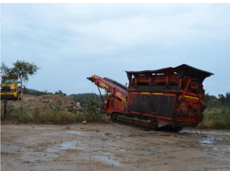
Crushing plant being placed on-site
