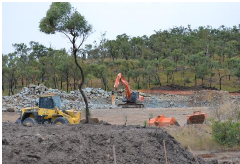
Powerlink bench construction
