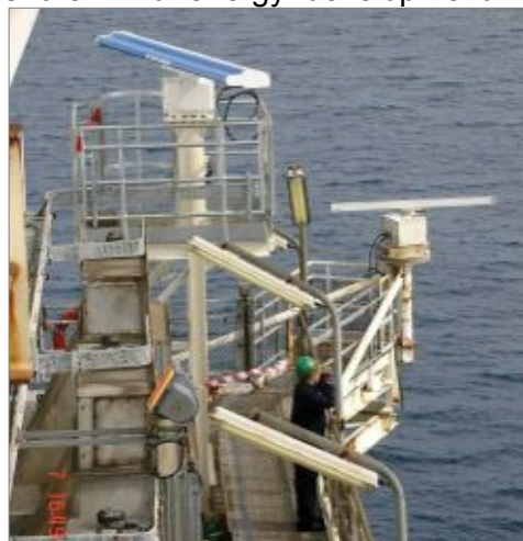
Furuno marine radar on the Talisman-Beatrice platform (top unit - blue); the MERLIN processor was installed in the equipment console to the left.
