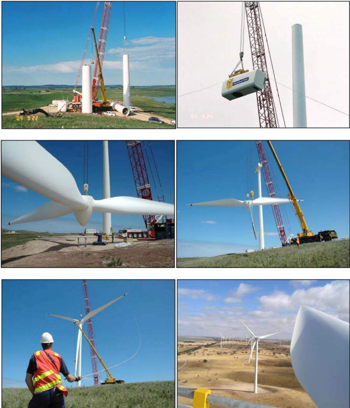
Plate 7 Illustrating typical activities during wind farm construction and installation.
