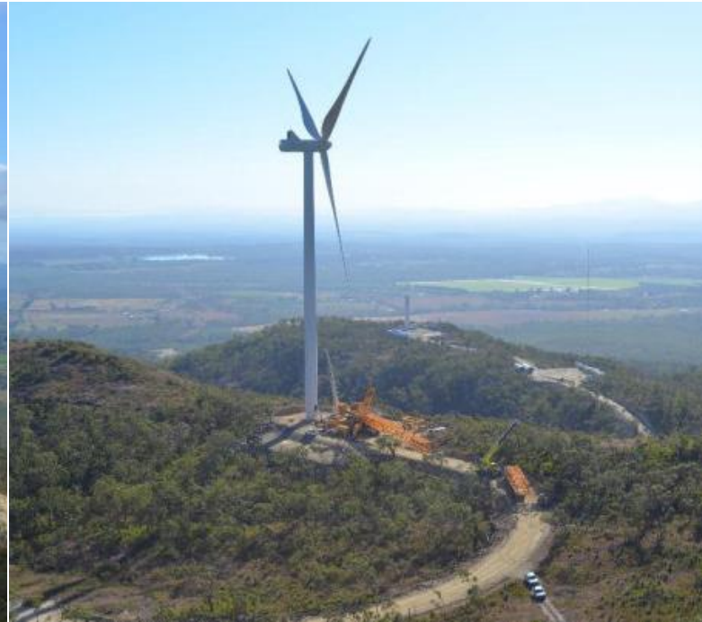
Complete install at WTG10
