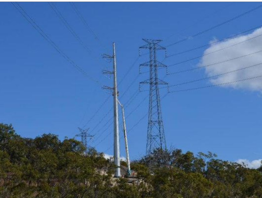
Cut-in and transfer works on Powerlink Transmission line
