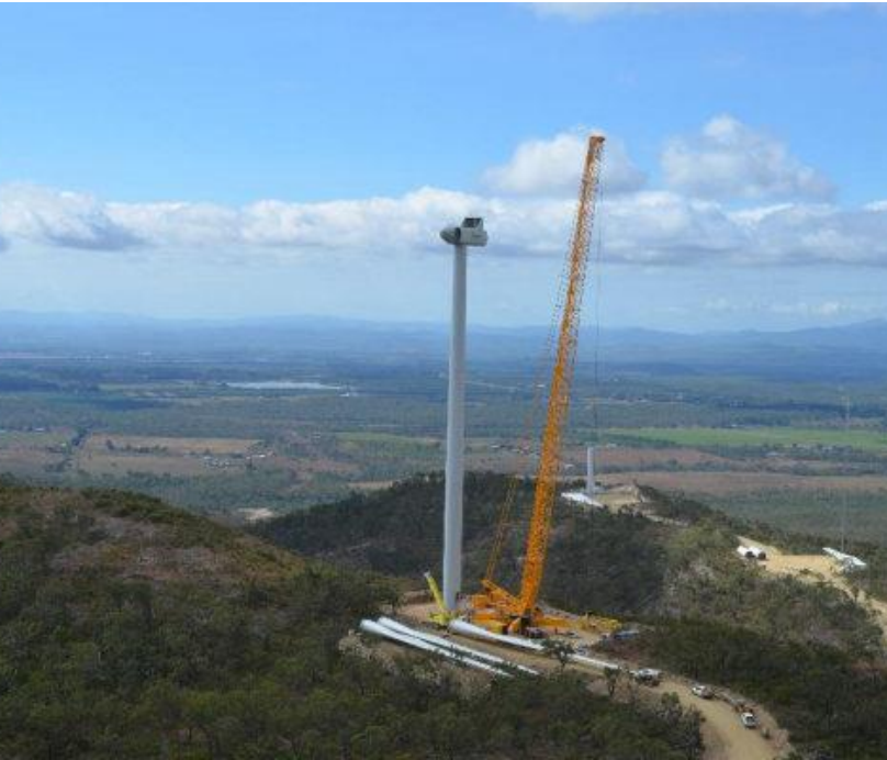
Tower install at WTG10
