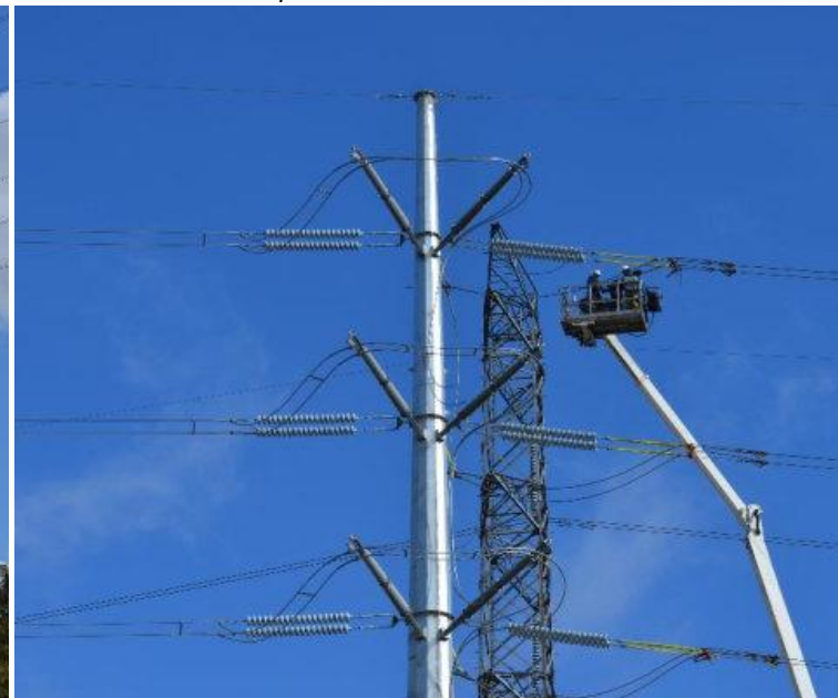
Termination of conductors on new pole
