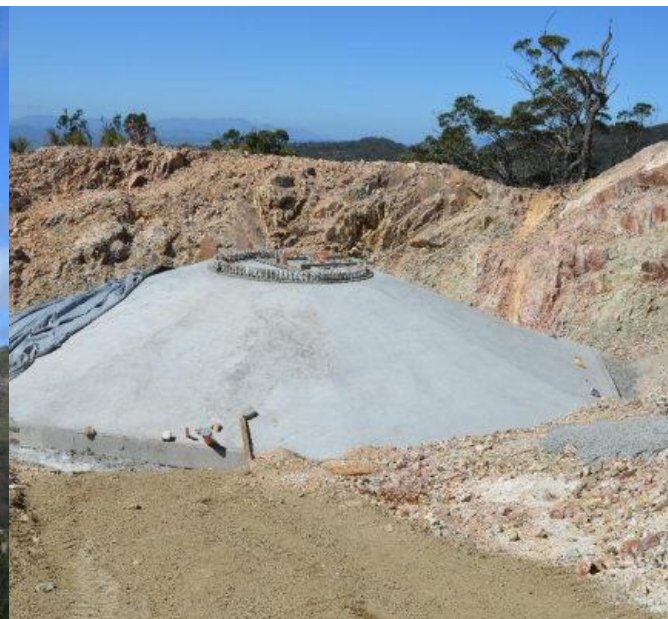
Final foundation – WTG33
