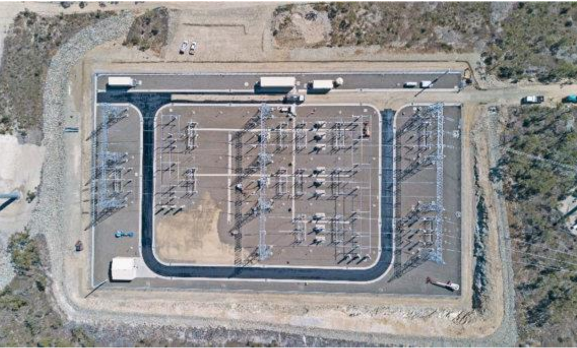
Aerial view of Powerlink Switchyard
