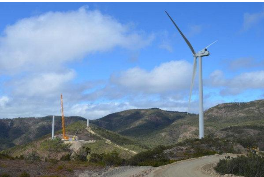
Installation at WTG19 and complete WTG20
