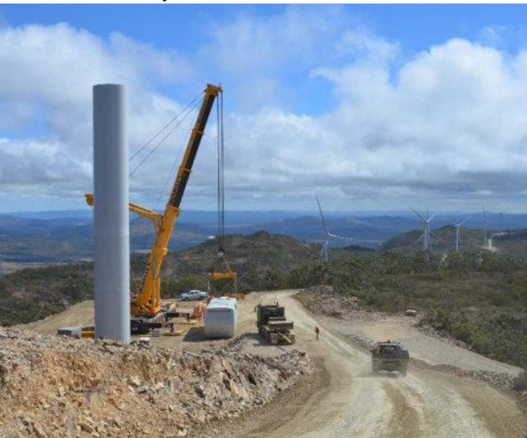
Installation work at WTG31
