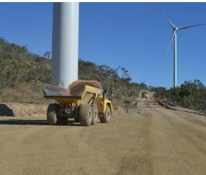
Road capping with cable trench on right verge
