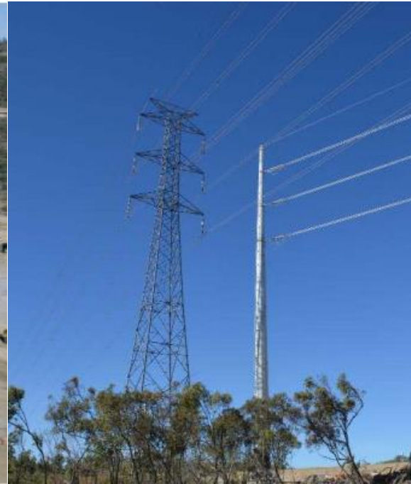
New power pole ready for connection
