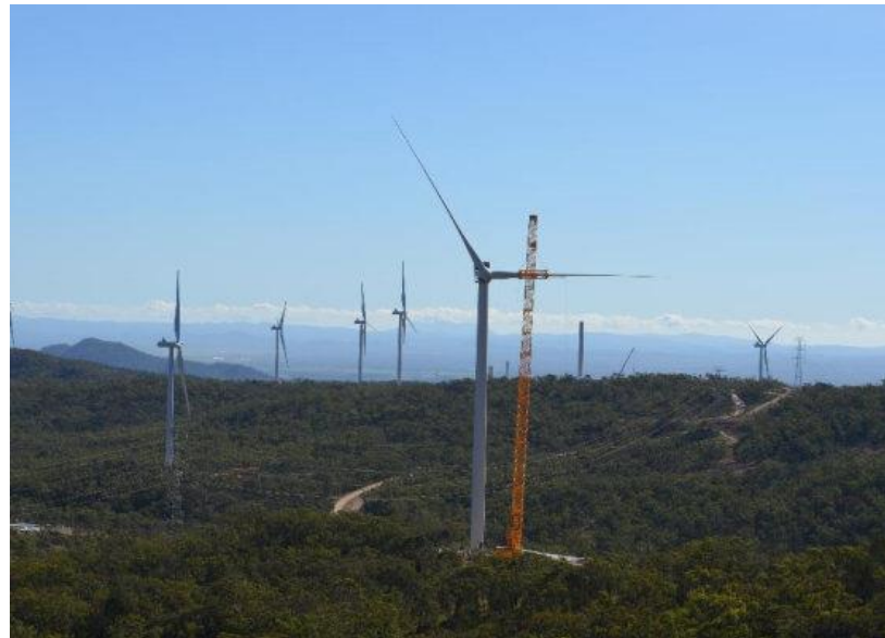
Blade install at WTG25
