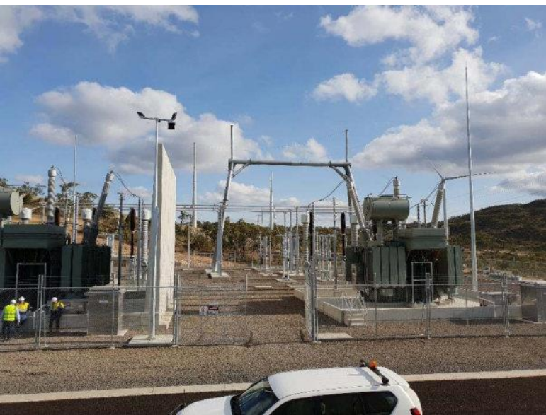
Wind farm substation nearing completion
