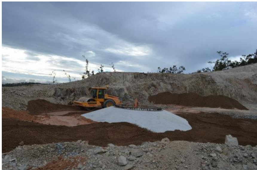
Backfilling of foundation at WTG27
