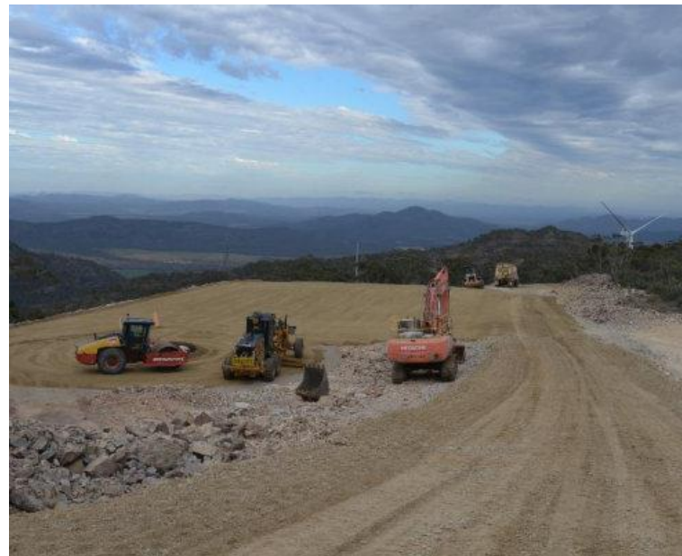
Completed hardstand at WTG31
