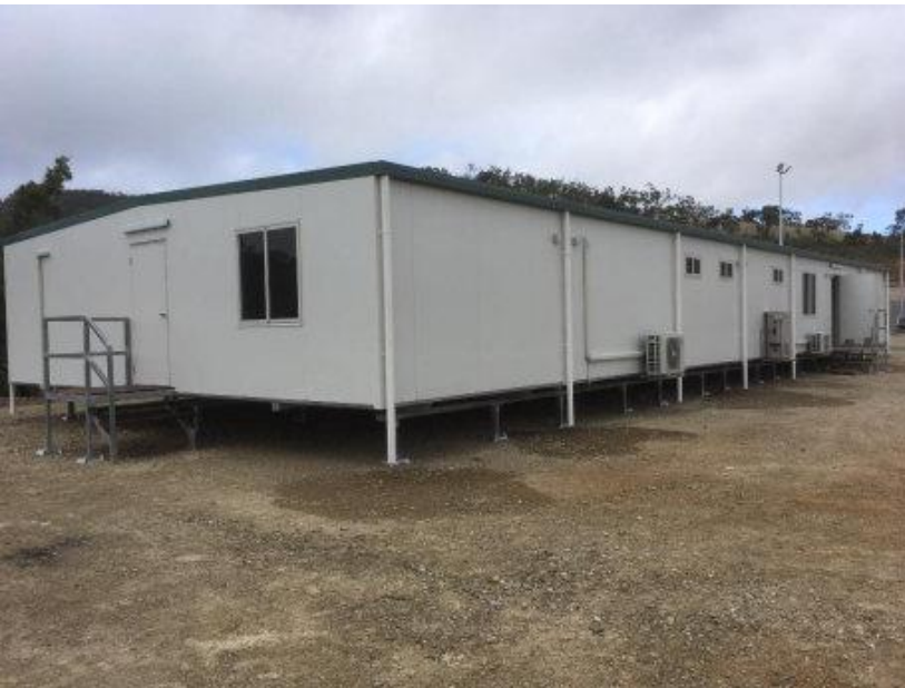
Operations and Maintenance Building
