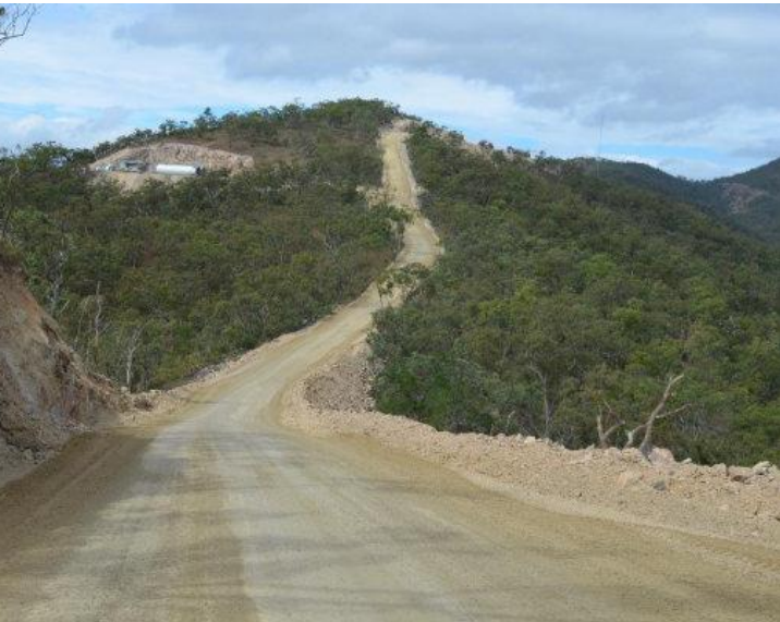
Access Road to WTG 19-20
