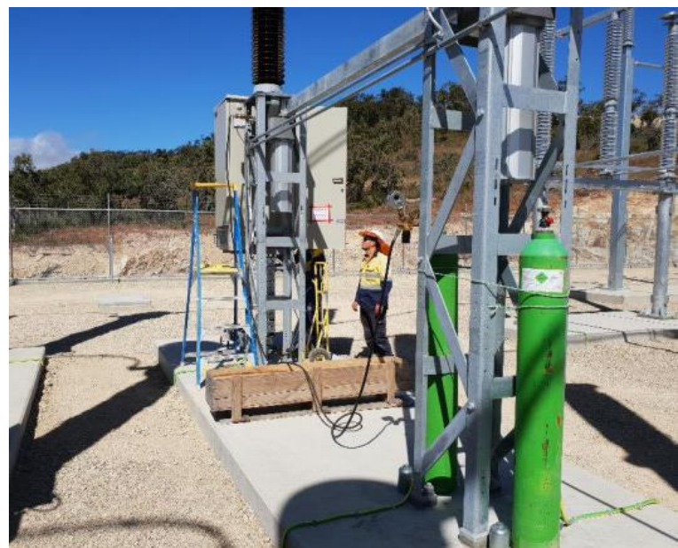
Install works continue at wind farm substation
