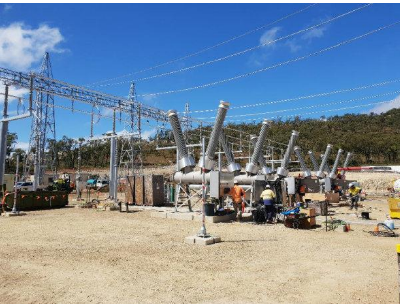
Install works continue at Powerlink switchyard
