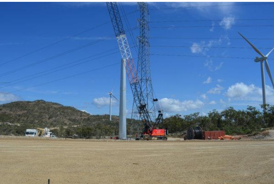
New transmission line pole being installed at Powerlink switchyard
