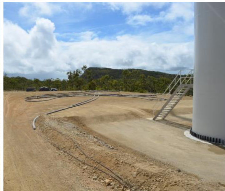
Cabling install complete
