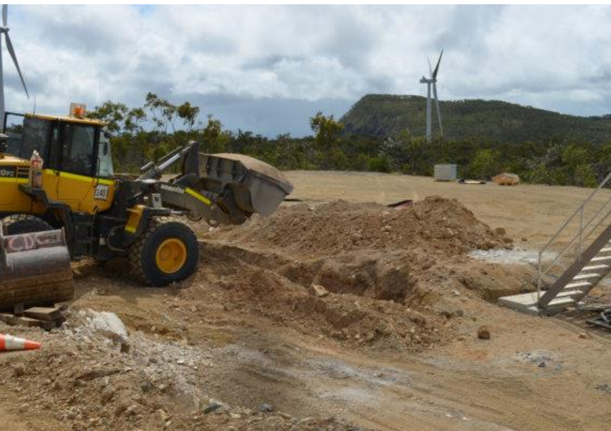
Backfilling of cable trench at WTG47
