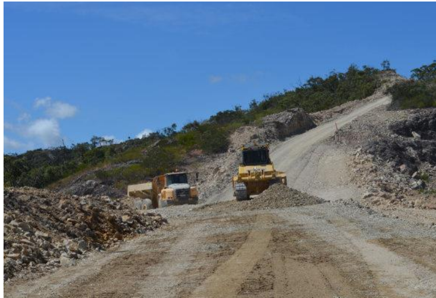
Access track to WTG31
