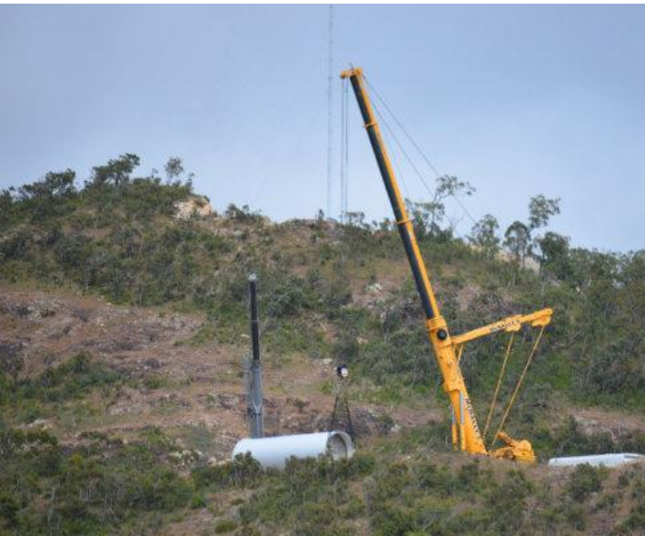
Base section install at WTG10
