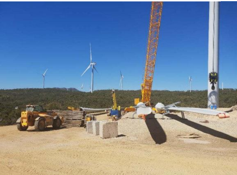
Blade installation preparation at WTG 50
