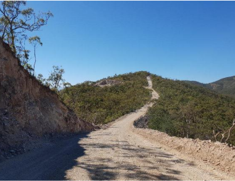
Access track to WTG 19 - 20
