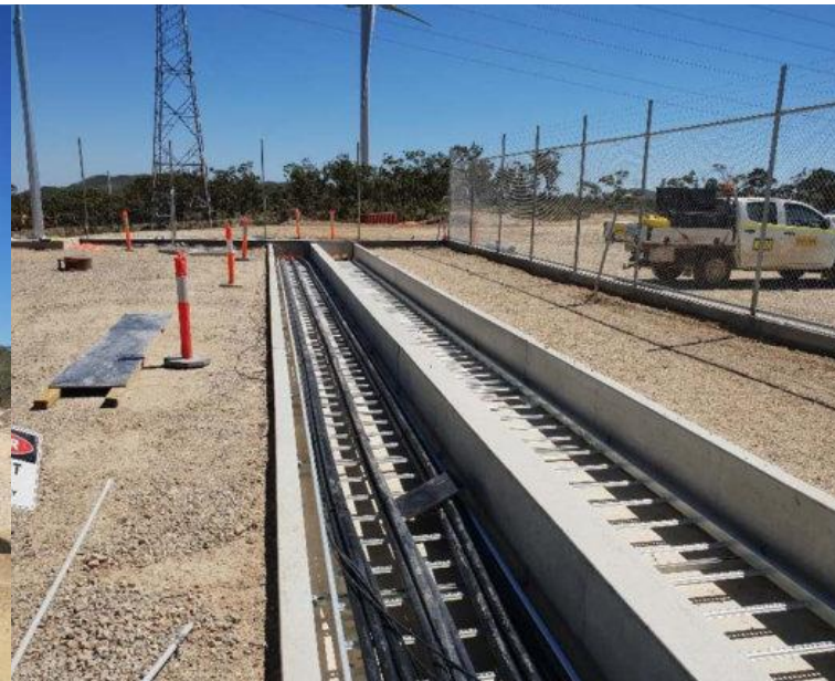
Collector trenches in wind farm substation
