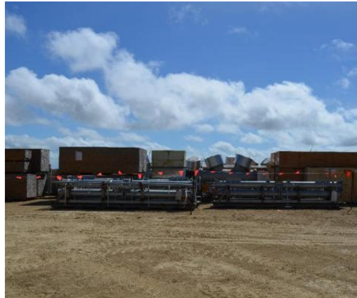
High Voltage equipment for Powerlink Switchyard
