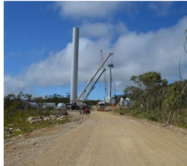
Blade unloading at WTG47
