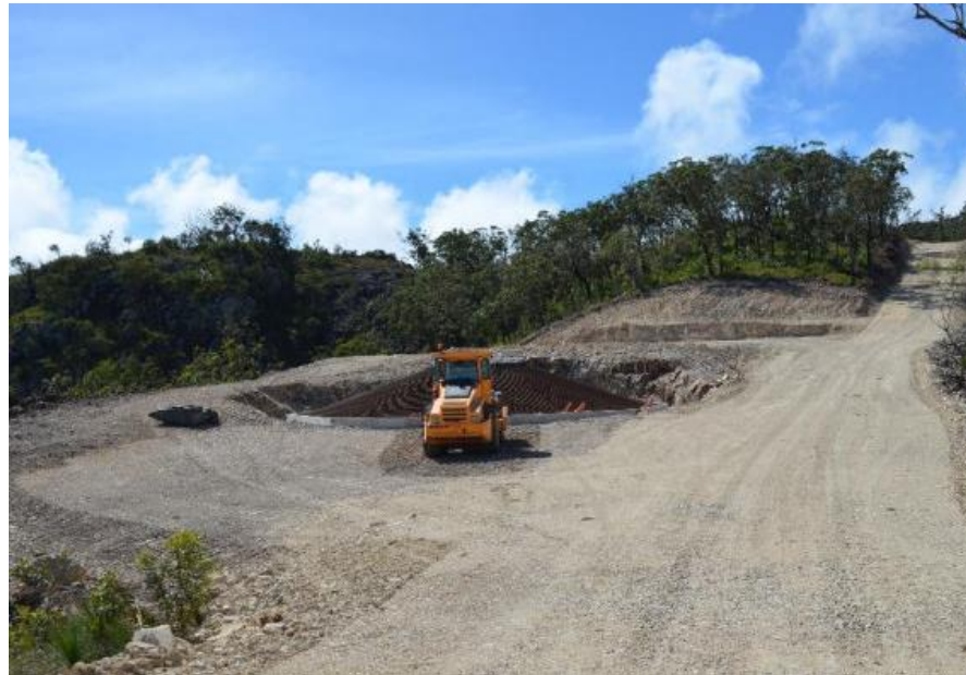
Road and Hardstand at WTG32
