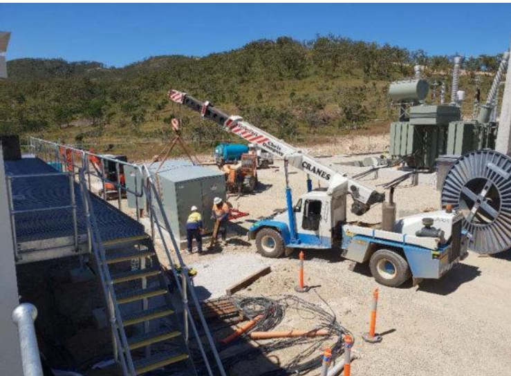
Wind Farm substation components being placed
