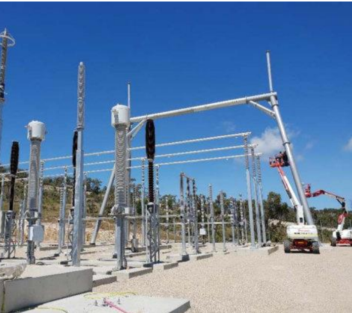
Landing gantry at wind farm substation
