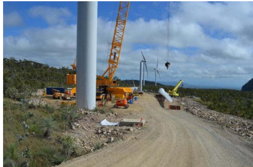
Installation at WTG43
