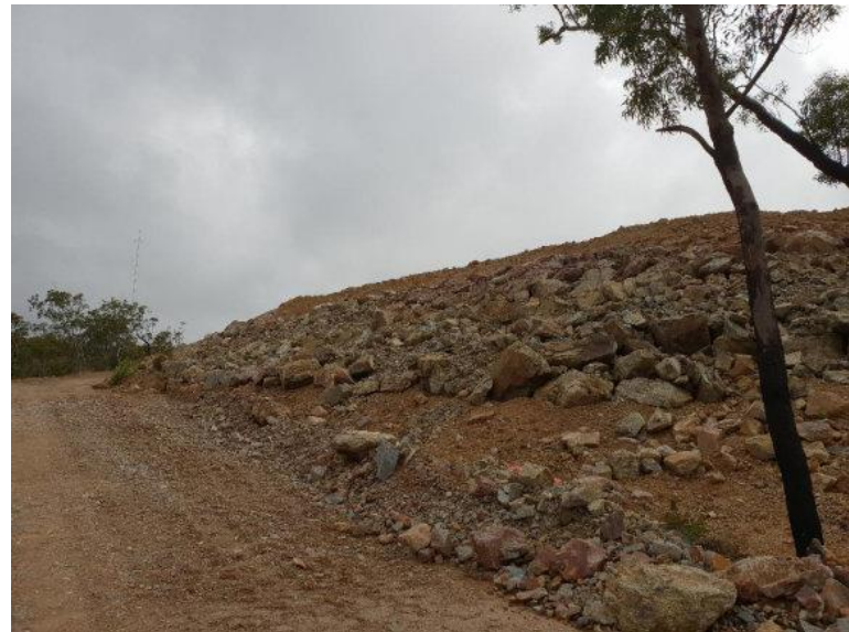
Rock armouring of batter slope at WTG19
