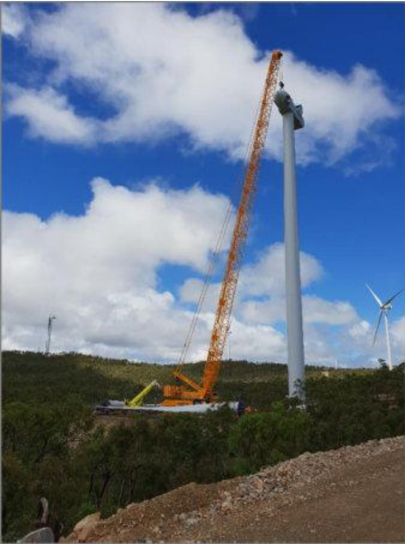
Hub installation at WTG51
