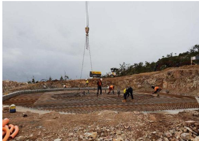
Placement of base reinforcing at WTG31
