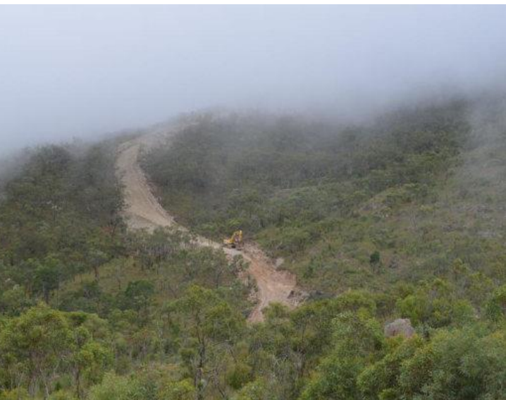
Road construction to WTG27
