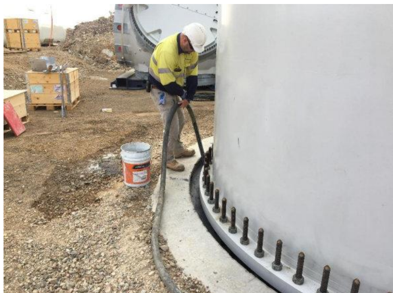
Grouting of base tower section
