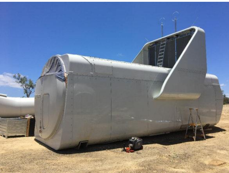
Turbine Nacelle ready for installation
