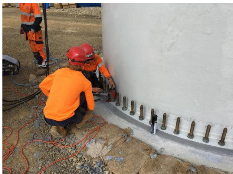
Bolt tensioning of base section
