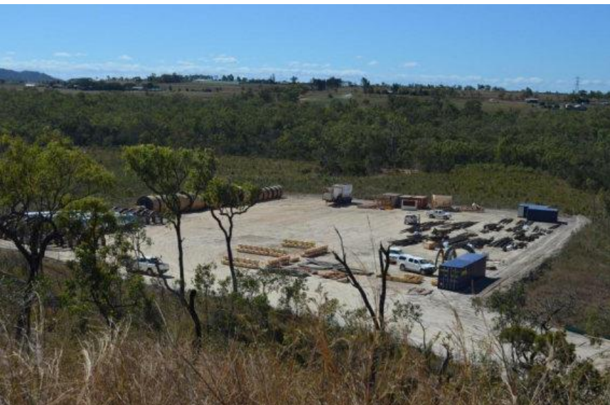
Lower Compound Laydown Area
