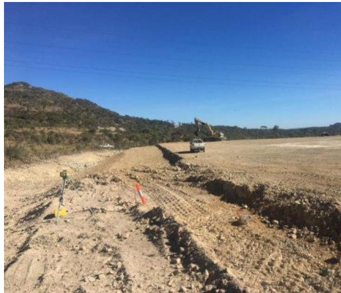
Capping of Powerlink Bench
