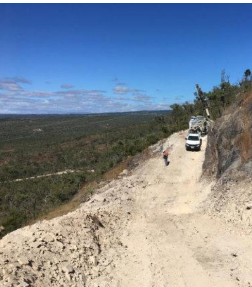
Construction of Site Access Road CH1300
