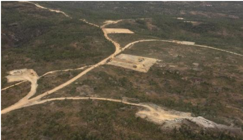
Aerial view of sites for WTG 2, WTG 3 and Upper Laydown Areas
